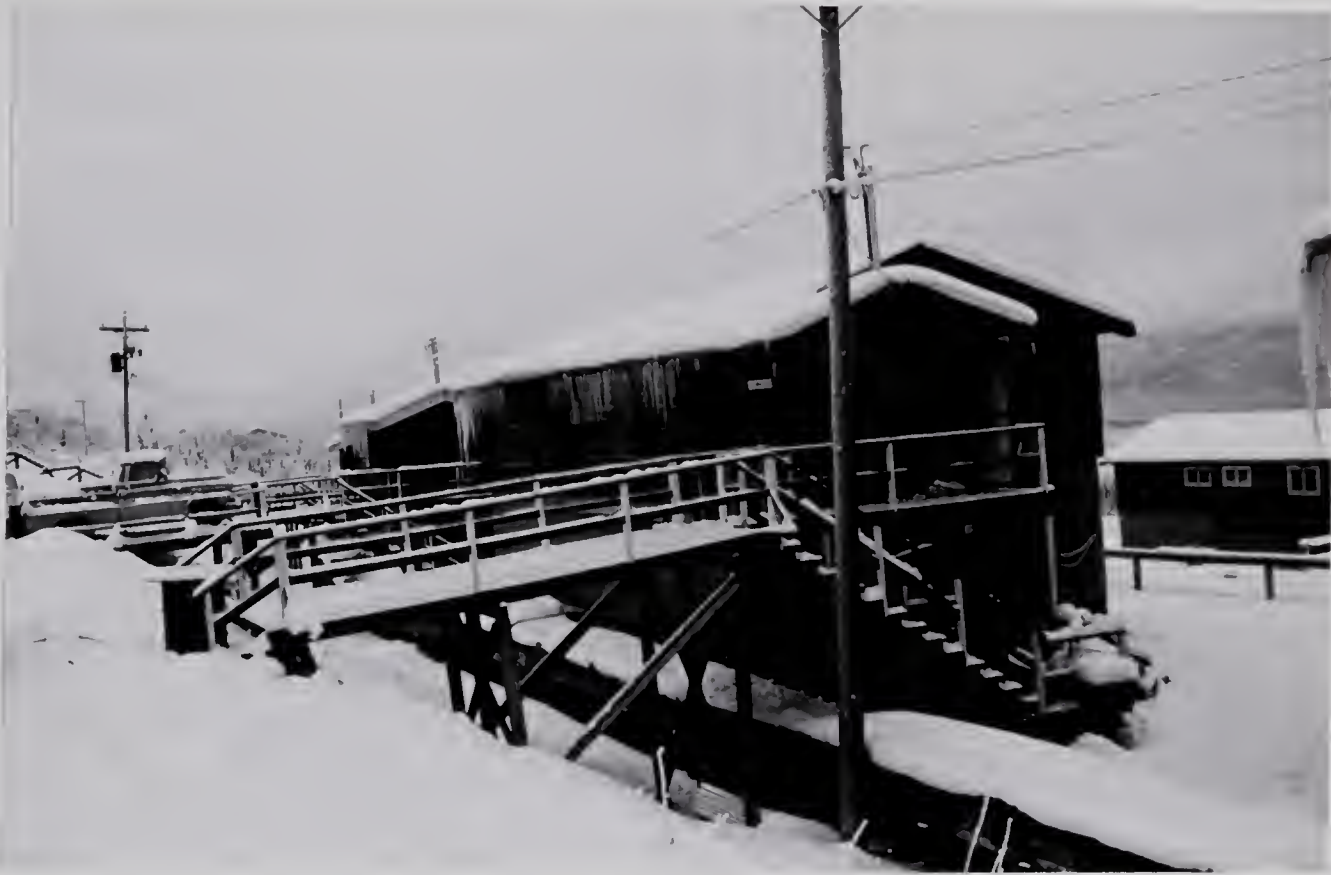
Plate 3. A new house in Elsa. The utilidor is beneath the walkway. (November 15, 1971).
